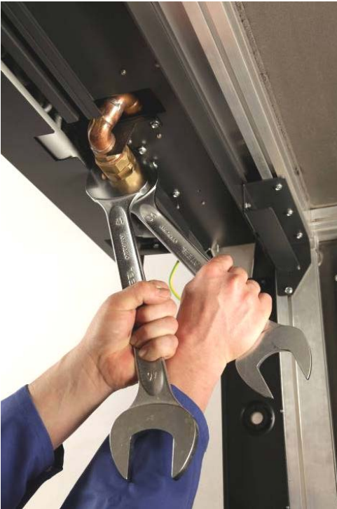
Figure 20 Tightening the union nuts
