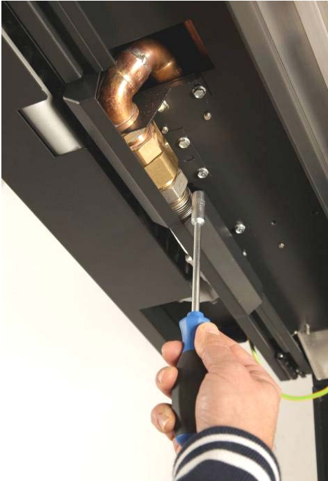
Figure 23 Attaching the swivel joint covers
