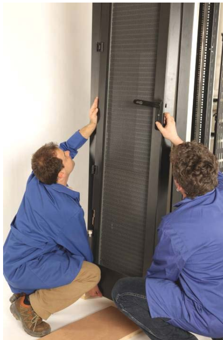
Figure 16 Installing the door
