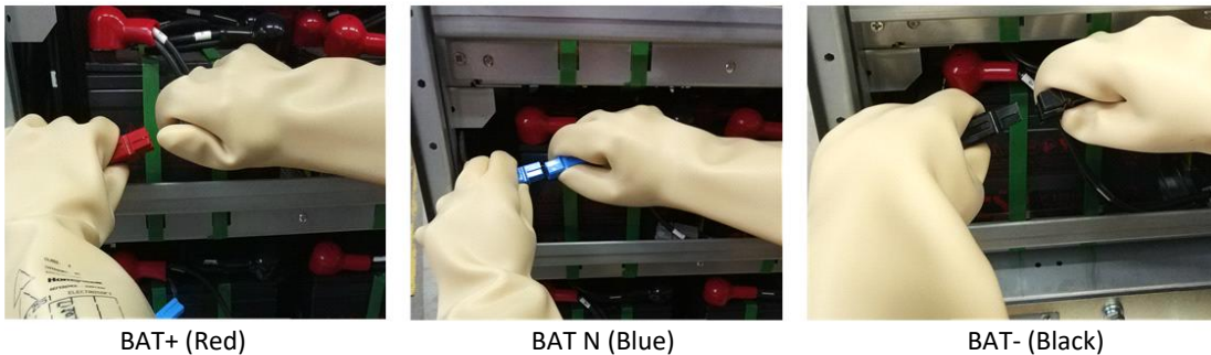
Figure 3-2 Connecting battery internal terminals
